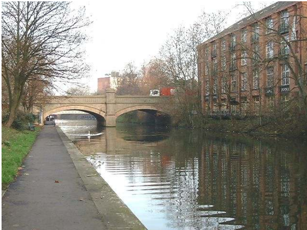
No. 21 The Newarke is a Grade II listed bridge over the Grand Union Canal
