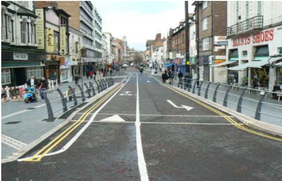
New carriageway/footway construction at Granby Street (2010)
