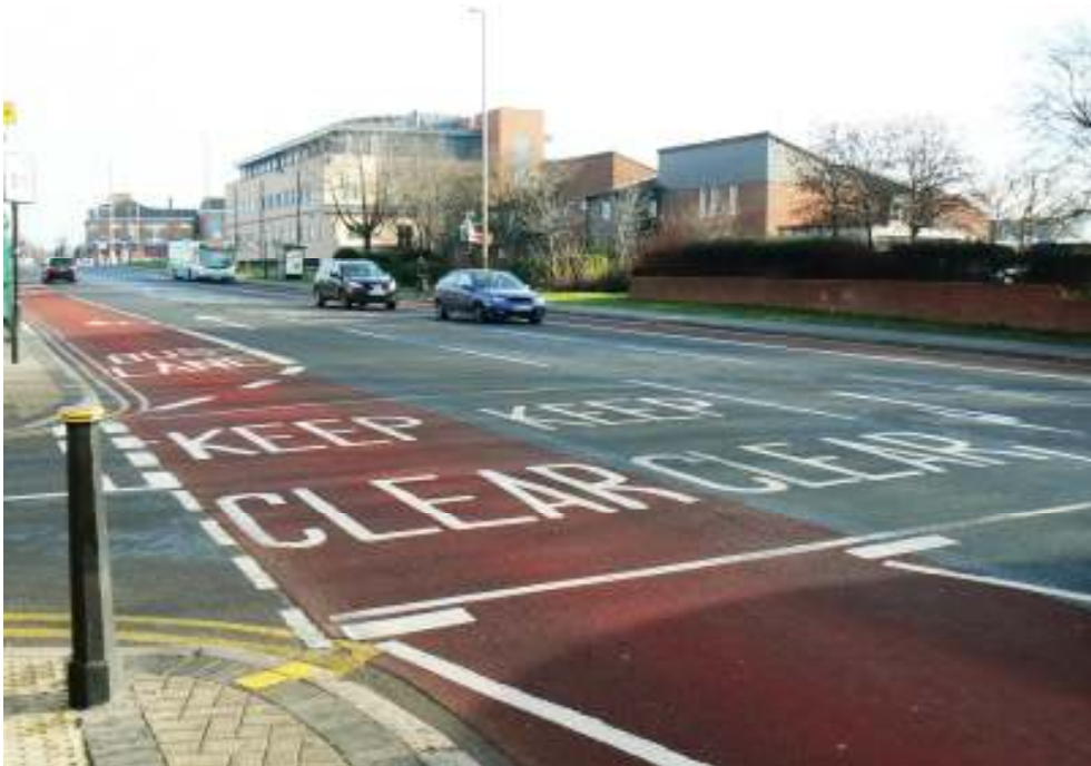
Integrated transport project on Humberstone Road (A47) completed 2010, resurfacing to road and footways, new bus lane and new anti-skid surfacing
