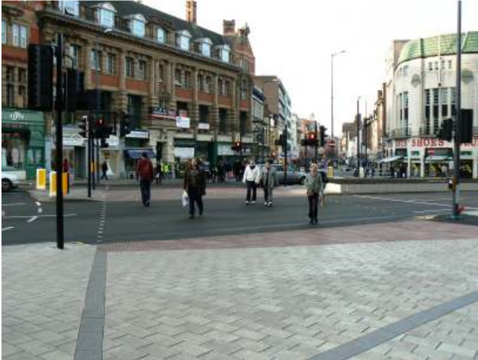
Super crossing at the junction of Granby Street and St Georges Way funded by Growth Point Funding and ERDF (European Regional Development Funding) - work completed 2010, resurfacing to road, new block paved footways, and controlled crossing.
