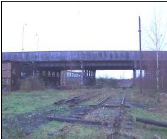
Pre scheme photo looking towards the elevation "Upperton Road"
